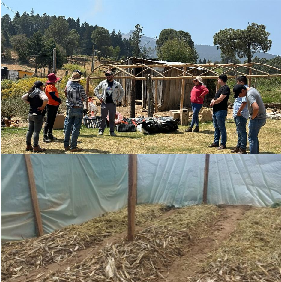
Figure 3. Installation of tunnels with local materials.
